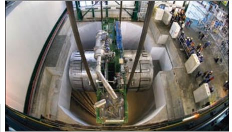
The central piece of CMS with the complete solenoid magnet just fits into the shaft down to the cavern 100 m below the surface.
