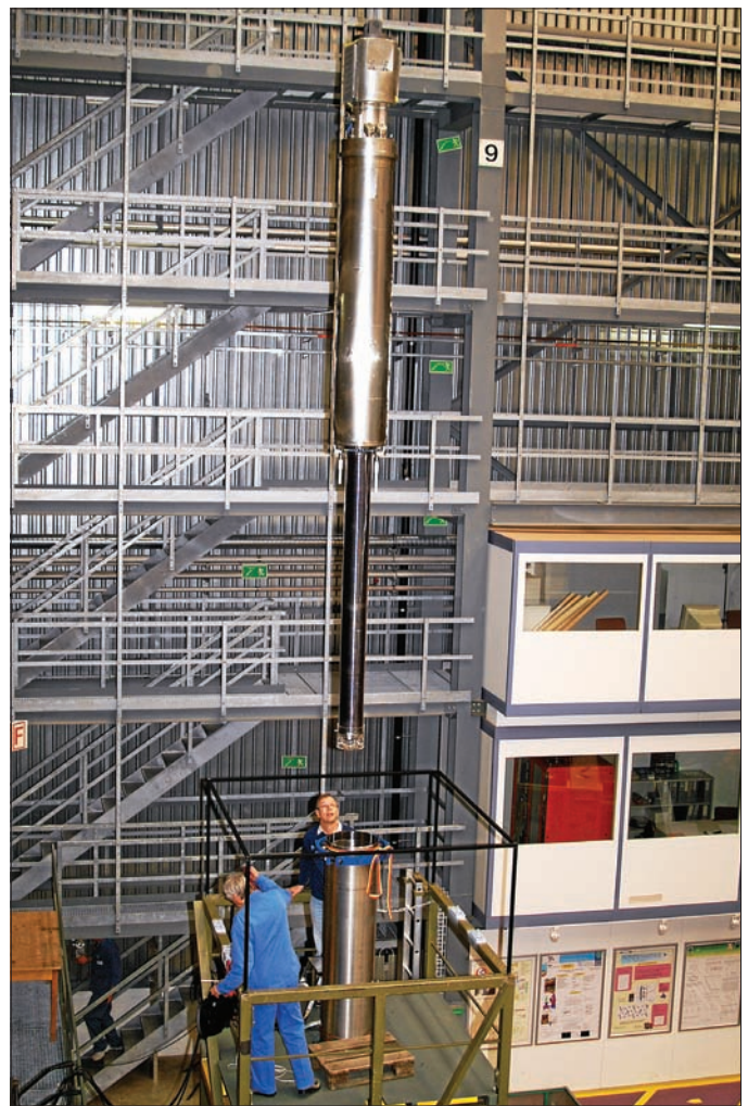
Installation of the 5 m long liquid-metal MEGAPIE target in the hall at the spallation neutron source, SINQ. (Courtesy PSI.)
