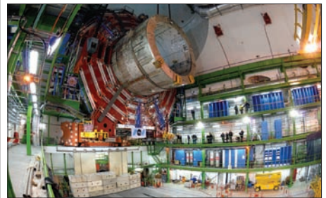
The piece emerges into the cavern after descending at a rate of about 10 m an hour.
